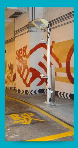
By using the vehicle License Plate as the primary identifier for the parking application, the project answered the challenges raised by dense city parking, as it audits and controls the parking revenues from one central location. In addition it provides a centralized service solution for the many residents of Hong Kong with easy and accurate parking subscriptions and discounts in their areas of residence.
